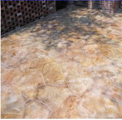
Completed resurfacing of patio.
