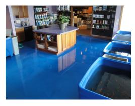
The first step is to put down a primer, which is typically a dark color such as black. Once that dries, simply apply a 20-mil spread of Aurora and wait approximately five to 10 minutes for the material to self-level. Once the time has passed, trowel, squeegee, or even blow the epoxy around the floor. This will redistribute the mica, creating the metallic look. Also, as the material settles, the dark primer shows through in the higher spots on the floor, creating additional visual depth.
