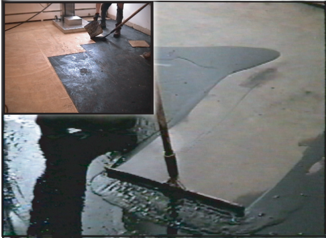
Remove asbestos mastic!
