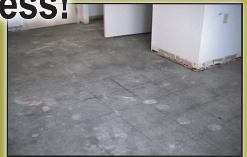
Ready to Resurface!
