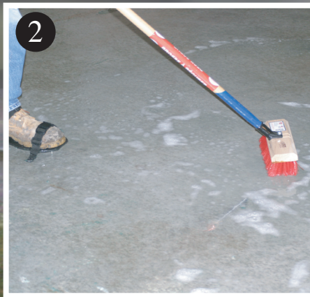
Scrub floor with degreaser
