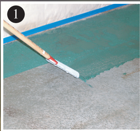
Scraping softened epoxy floor paint
